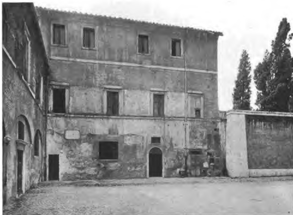
Fig. 96 — S. Lorenzo f.l.m. Convent, west wing from north with northeast corner of basilica maior left of drain pipe (Photo: Sansaini).
